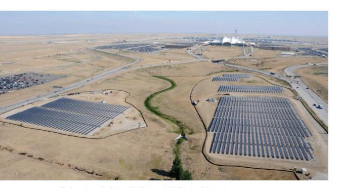
The Denver International Airport (DIA) features a 2 MW PV system. DIA is now host to a second 1.6 MW array system. (Denver International Airport/PIX18043)
