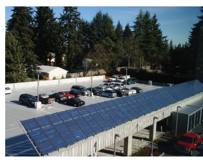
The City of Shoreline, Washington, installed a 20.2 kW solar electric system on top of the City Hall parking garage. The system uses Washington-made solar modules from Marysville-based Silicon Energy. (City of Seattle/PIX18074)
