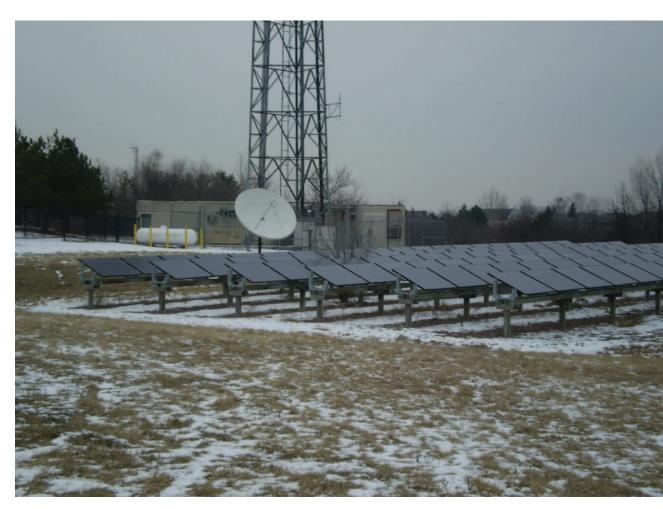
The 100 kW ground-mounted PV system is co-located with an electrical substation in Ann Arbor, Michigan. (Vipin Gupta/PIX179326)
