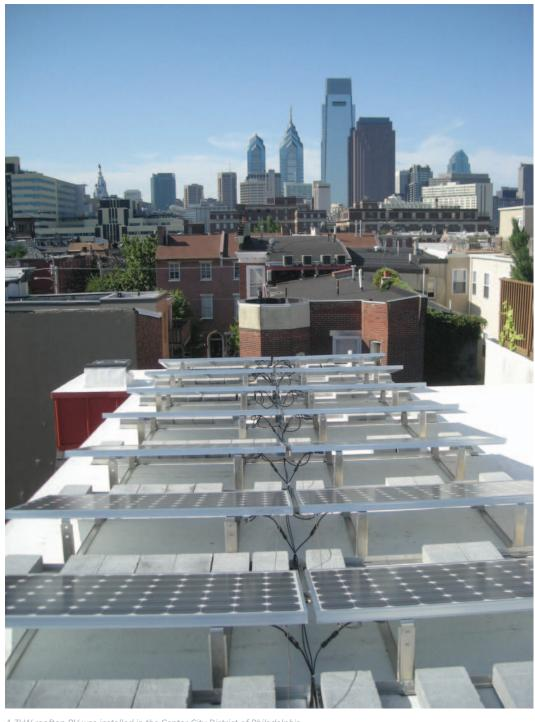
A 3kW rooftop PV was installed in the Center City District of Philadelphia. (Mercury Solar Solutions/PIX18063)
